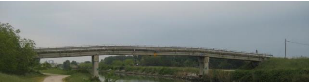
Bridge n.2: a pre stressed r.c. cantilevered bridge.
