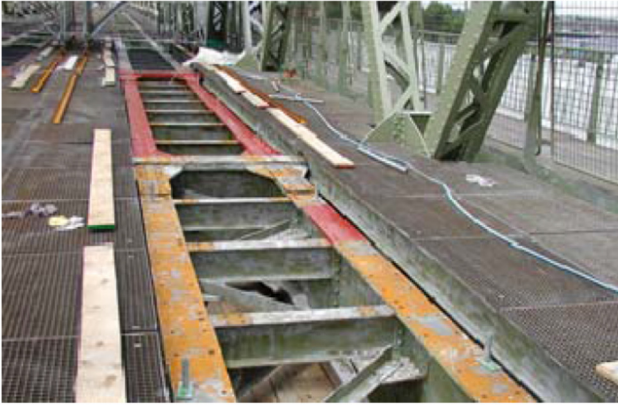
Removed bridge sleepers and New silent bridge® decks
