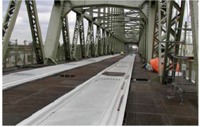
Removed bridge sleepers and New silent bridge® decks
