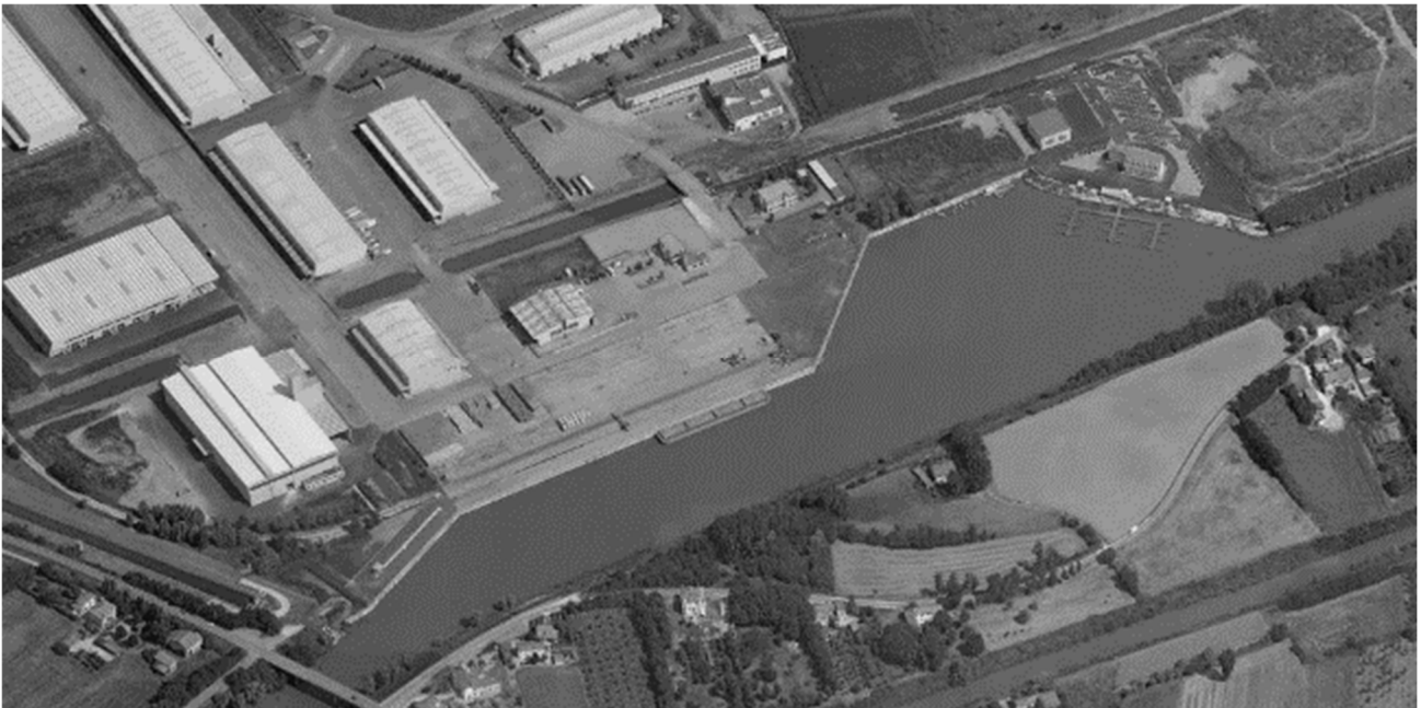
The quay walls along the Milano-Adriatic sea waterway.
