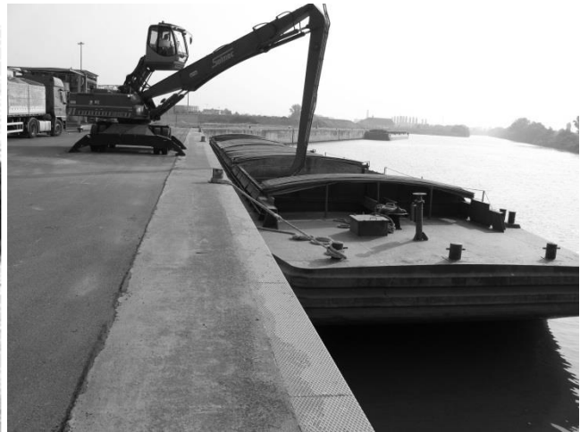
Local quay surveillance: road sinking (left), undamaged embankment (right).
